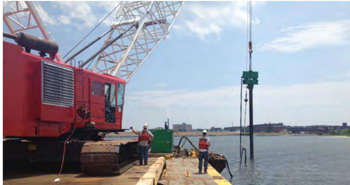
**Figure 5. Pile Probe Exploration for Obstructions in Progress**
