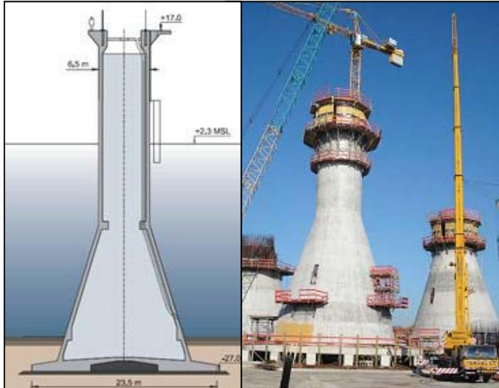
**Figure 8: Gravity Base Foundation<sup>12</sup>**
