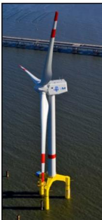
The tripile foundation is also a relatively new adaption of the traditional monopile foundation. Instead of a single beam, three piles are driven into the seabed, and are connected just above the water's surface to a transition piece using grouted joints. This transition piece is connected to the turbine tower's base. The increased
