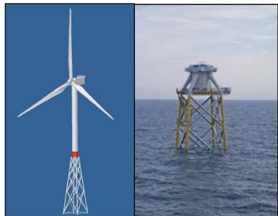
**Figure 9: Jacket Foundation<sup>13-14</sup>**
