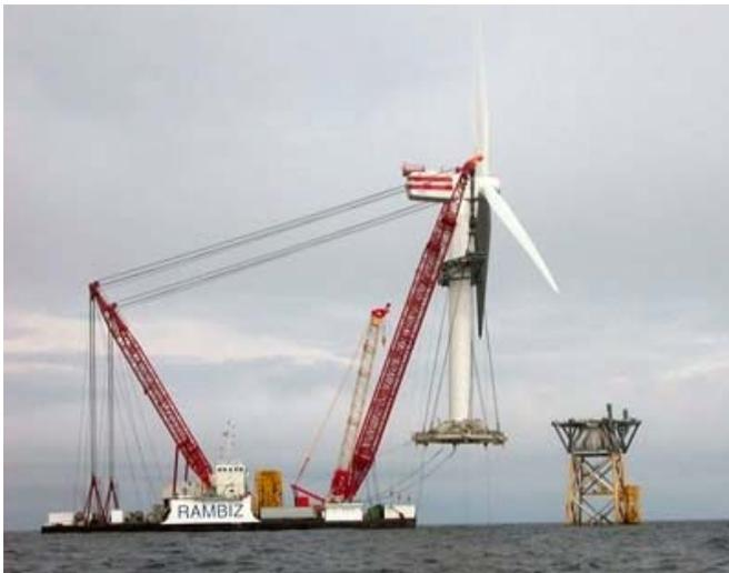
Figure 17: Heavy Construction Vessel Installing Wind Turbine on Jacket Foundation<sup>26</sup>
